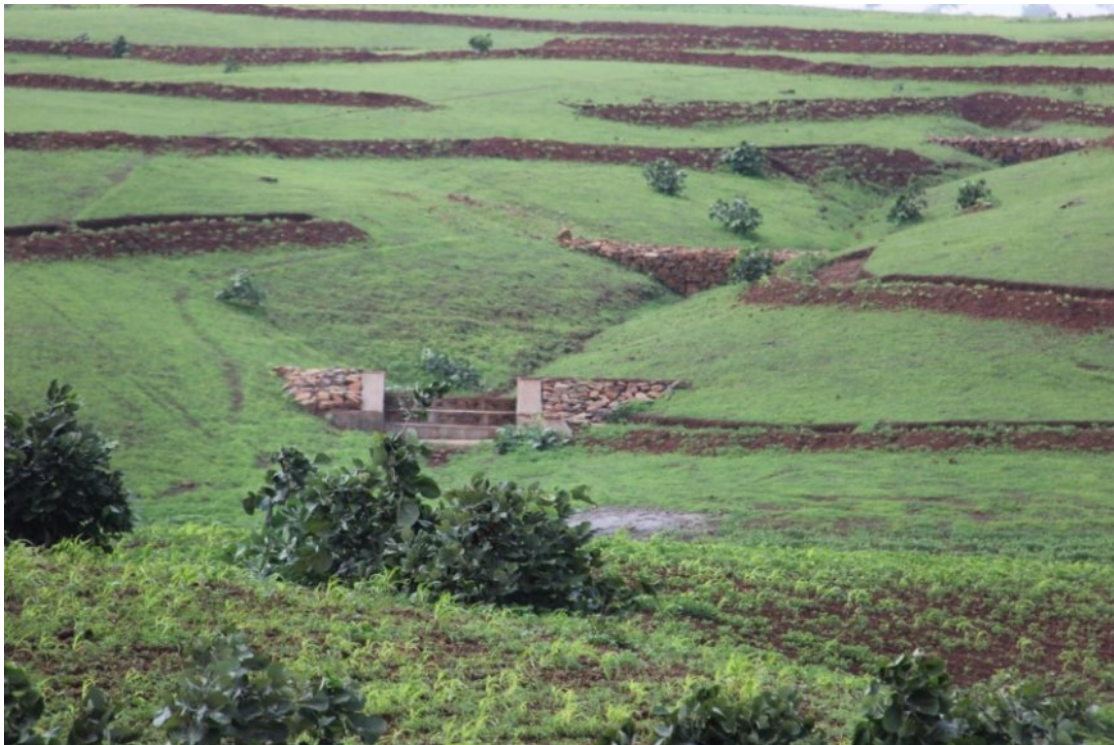
SWS PATAN SOILWORK & GABION YEAR 2014-15
